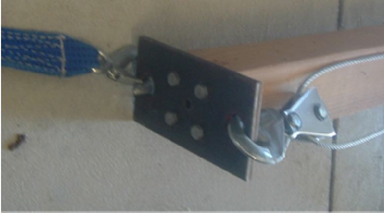
The steel plate on top of the derrick post.
