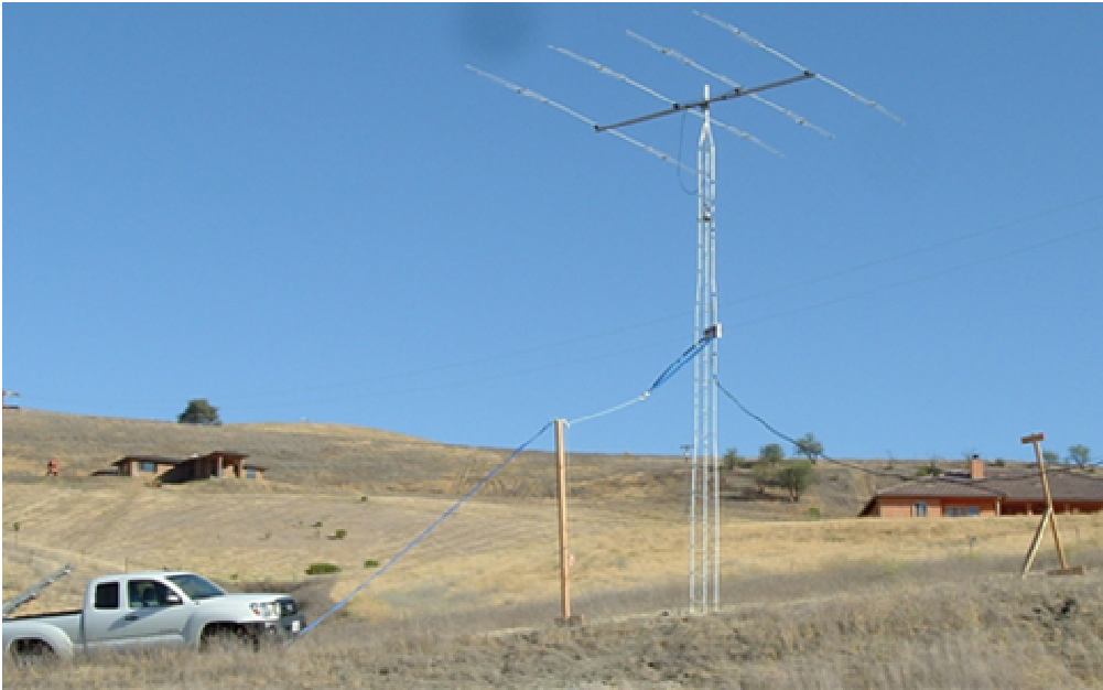
The set up after raising. The 10' 2X4 support is at the right.
