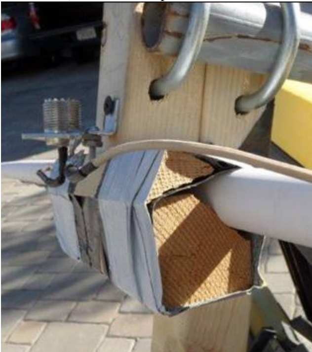
End view (note use of a split-off 2X2 corner to make a clamp) showing plenty of duct tape.
